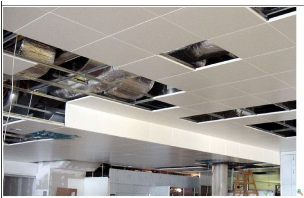
Figure 5: Clamped cassette ceiling during installation (Source: LSMW GmbH, D-90408 Nürnberg, www.lsmw.de )
